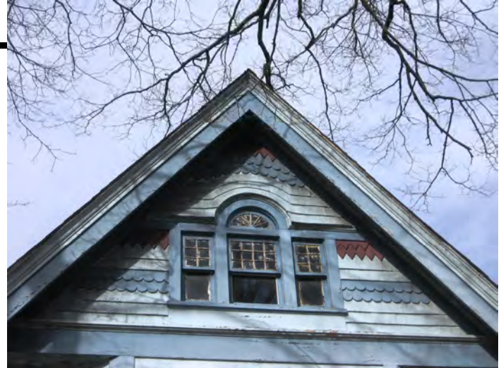
Paint protects wood and highlights ornamental features such as the decorative wood shingles and Palladian window at 618 Ingleside Avenue.
