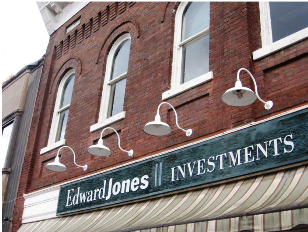
These "gooseneck" light fixtures are appropriate designs for the building at 10 S. White Street.
