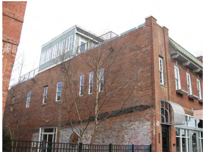
This rooftop addition is appropriate since it is recessed from the main façade, of limited height and not readily visible from the street.
