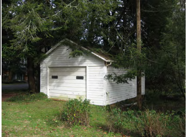
Historic wood frame outbuildings such as the garage at 508 Ingleside Avenue (above) and shed at 505 E. Madison Avenue (below) are important resources of the property.
