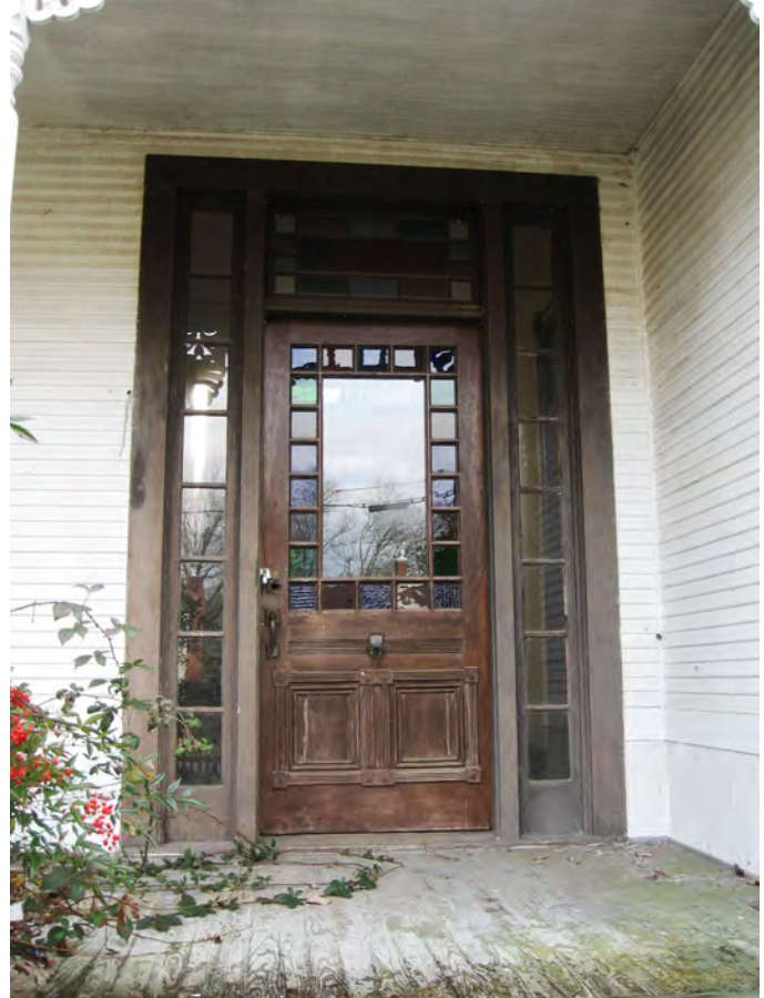
The house at 505 E. Madison Avenue has an original two-panel door with a single light bordered by decorative stained glass lights. The entrance also retains sidelights and transom.
