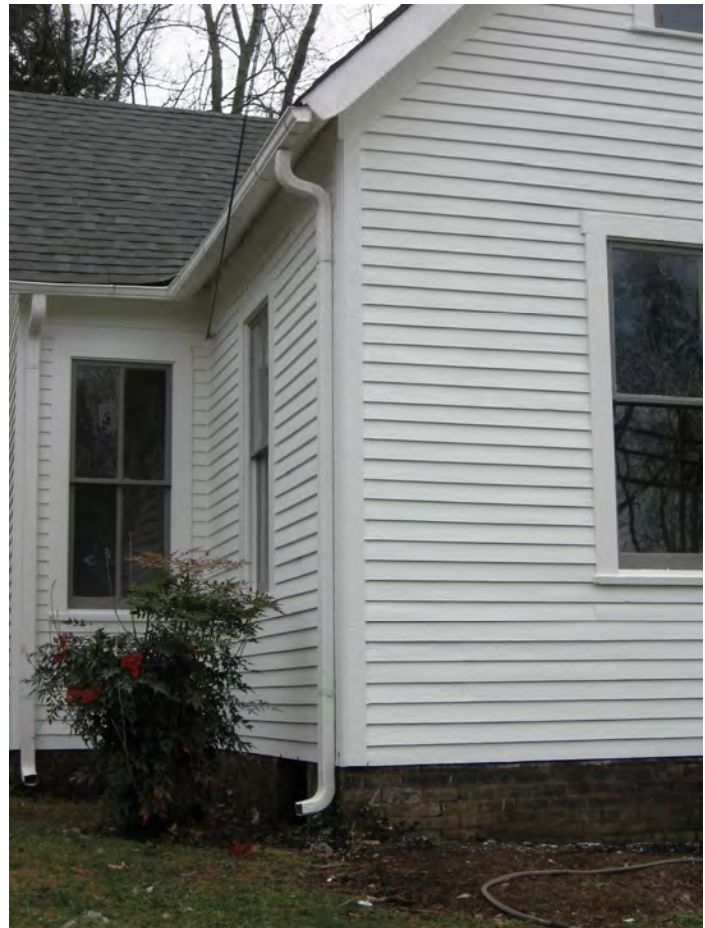
Example of an appropriate gutter and downspout at 601 Ingleside Avenue.
