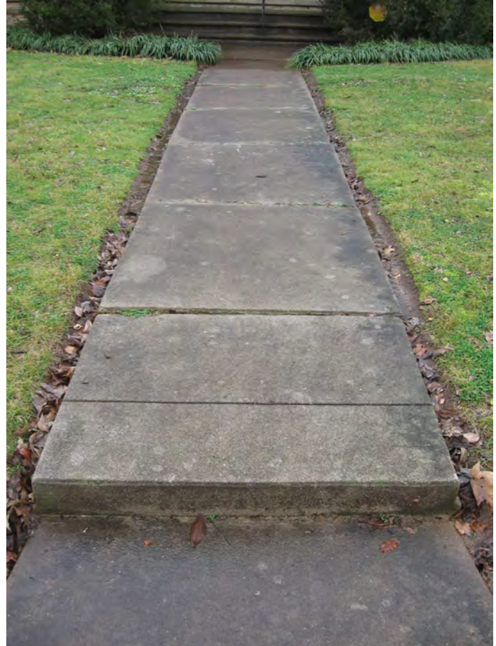
Retain and maintain original concrete walkways (612 E. Madison Avenue).
