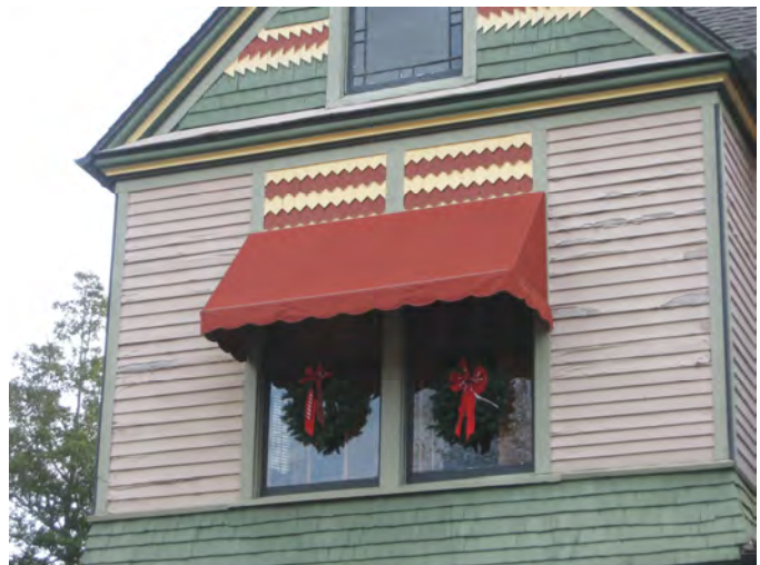
Window awnings can assist in lowering energy costs during warmer months.(419 E. Madison Avenue).
