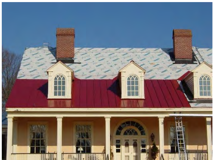
New metal roofs shall have crimping and spacing to match original metal roof designs of the dwelling's period.
