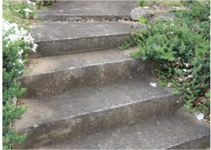
Preserve and maintain original concrete steps (701 N.
