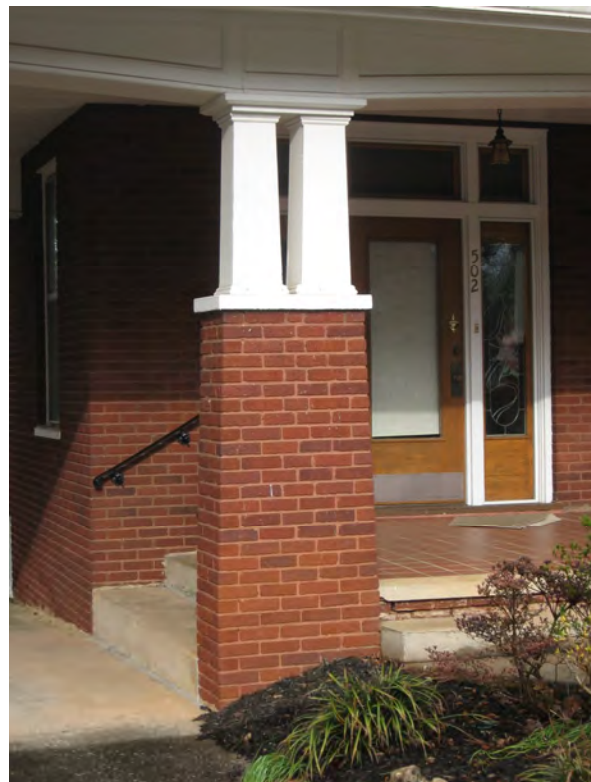
Unpainted masonry features such as porch columns should be left unpainted unless the brick is badly damaged or has numerous repairs (502 E. Madison Avenue).
