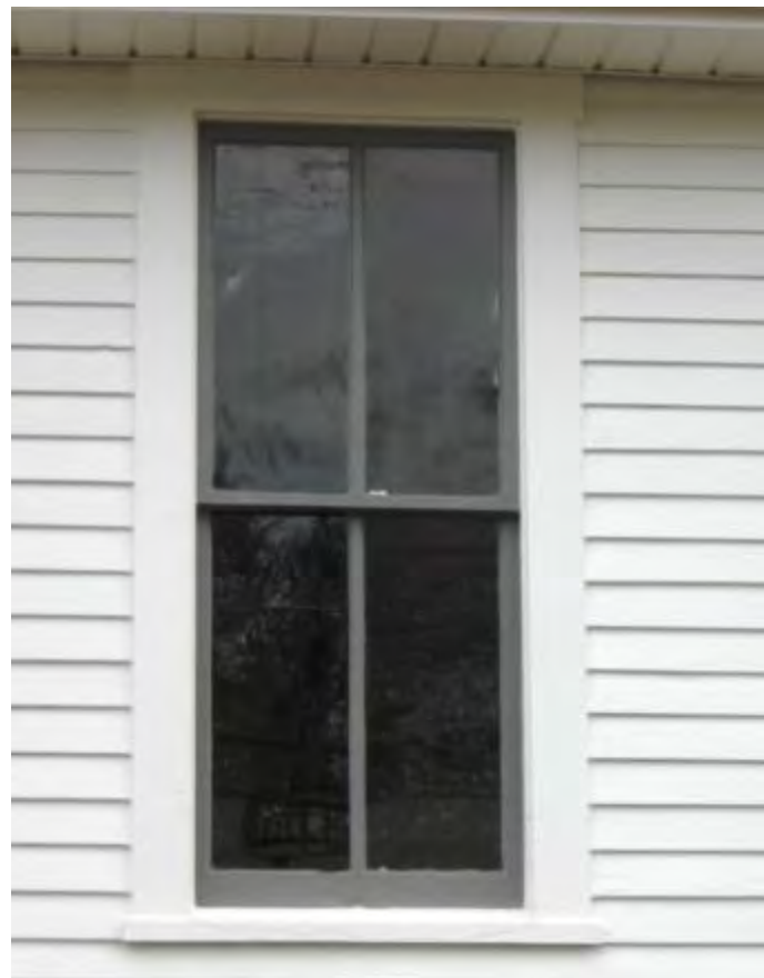
Original two-over-two, wood-sash windows help identify a dwelling's date of construction to the late 19th century (601 Ingleside Avenue).
