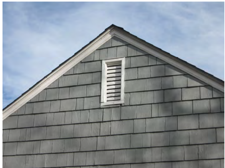
Retain and do not conceal original wood features such as the shingles in the gable field at 9 Walcon Lane.
