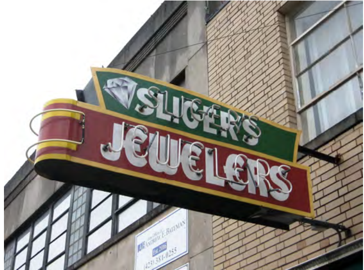
The business at 116 E. Washington Street has a restored vintage neon sign which should be preserved and maintained.
