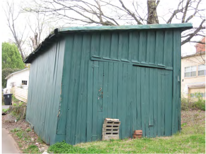
This early garage is distinguished by its board and batten siding and shed roof (600 N. Madison Avenue).
