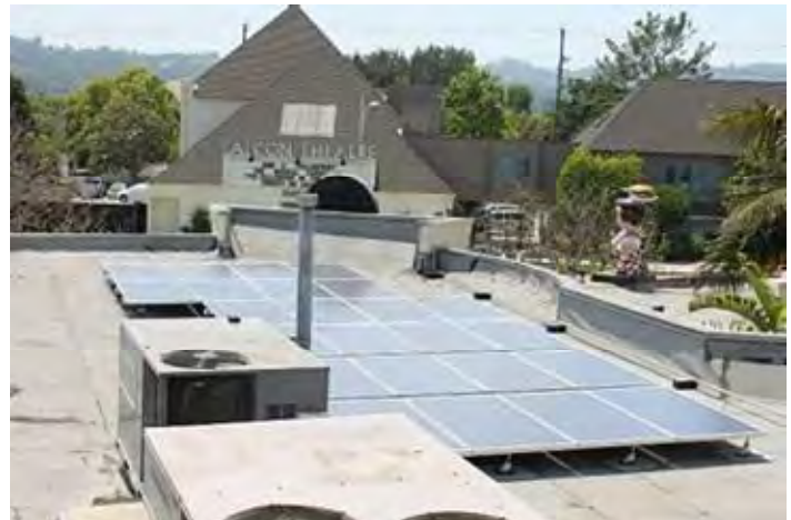
The installation of solar panels on roofs of commercial buildings is appropriate and encouraged. These panels are sited below a building's parapet wall and are not visible from the street.
