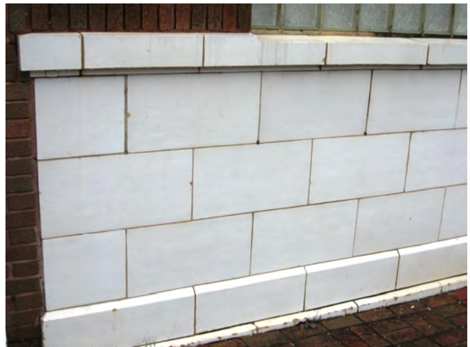
The frame bulkhead at 118 N. Jackson Street (above) and the glazed-tile bulkhead at 2 N. White Street (below) are examples of storefront surfaces that contribute to a varied texture in the commercial streetscape.
