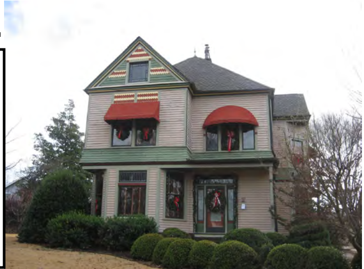
The irregular roof plan and components are character-defining features of the Queen Anne-style dwelling at 419 E. Madison Avenue.
