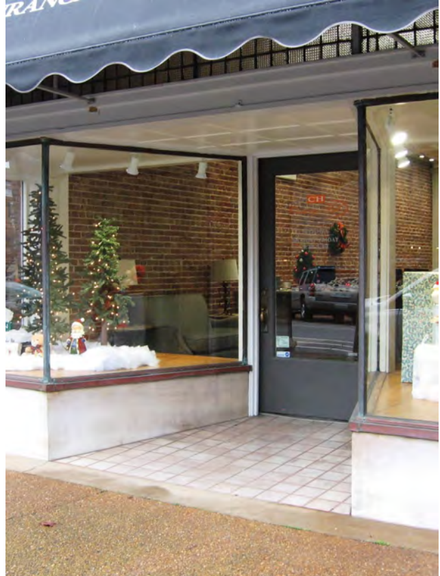
This original storefront at 110 E. Washington Avenue retains its recessed entrance and display windows and single-light door.
