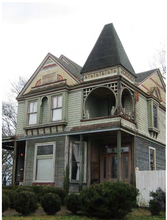
The Queen Anne style features an asymmetrical plan, corner tower, and wood trim details (511 E. Madison Avenue).
