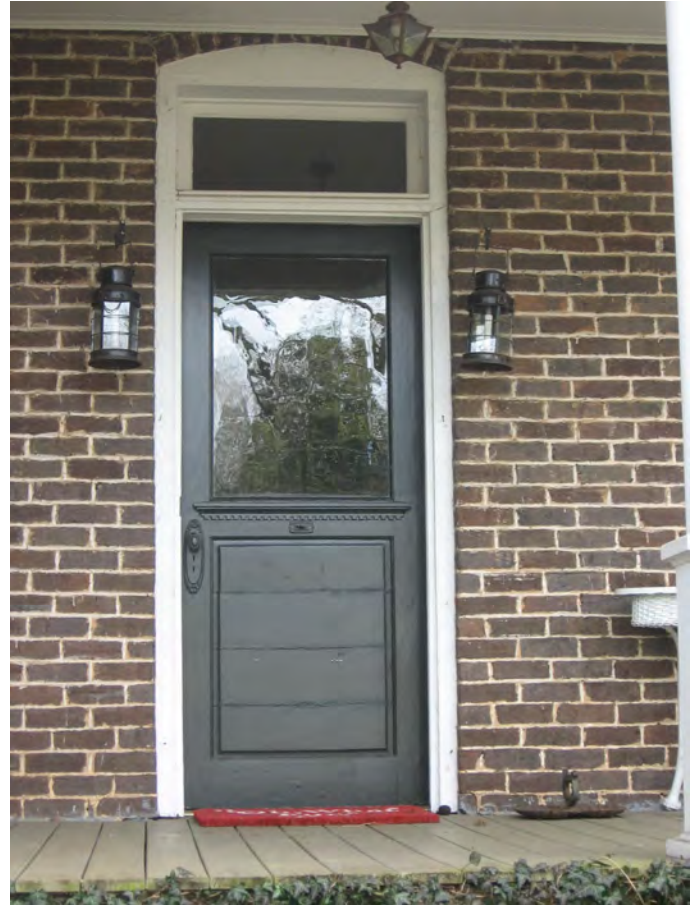
The entrance at 505 Ingleside Avenue has an original single-light, single-panel wood door, a single-light transom, and a simple arched surround.
