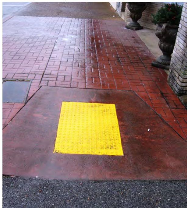
The city has undertaken a number of ADA-compliant efforts such as the sidewalk curbing at White and Hornsby Streets
