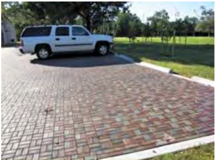
The City of Athens should consider the use of permeable paving surfaces for public parking lots to allow for absorption of water and less run-off into storm sewers.
