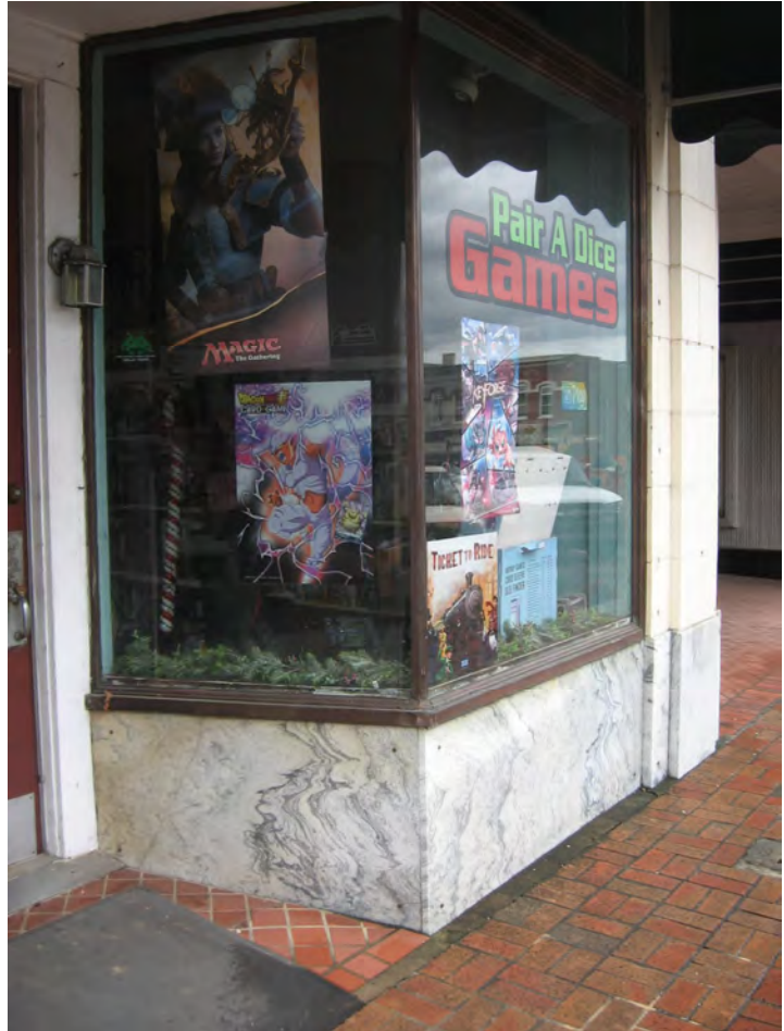
The marble paneled storefront at 2 E. Washington Avenue (above) and the Carrara glass accent courses below a pressed metal ceiling at 4 E. Washington Avenue (below) are examples of storefront surfaces that should be preserved.
