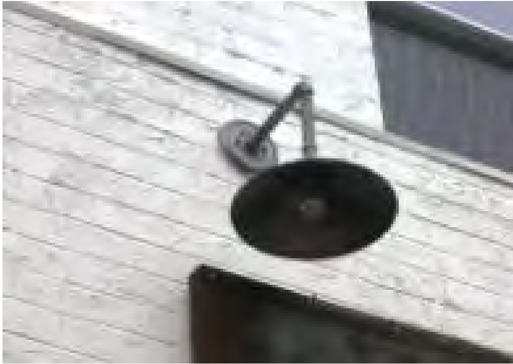
An appropriate fixture for illuminating commercial buildings and signs (6 E. Washington Avenue).
