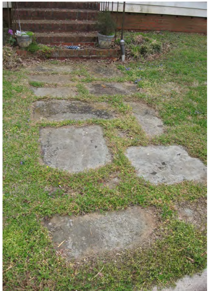
This random pattern stone walkway pattern should be preserved and maintained (710 N. Ingleside Avenue).
