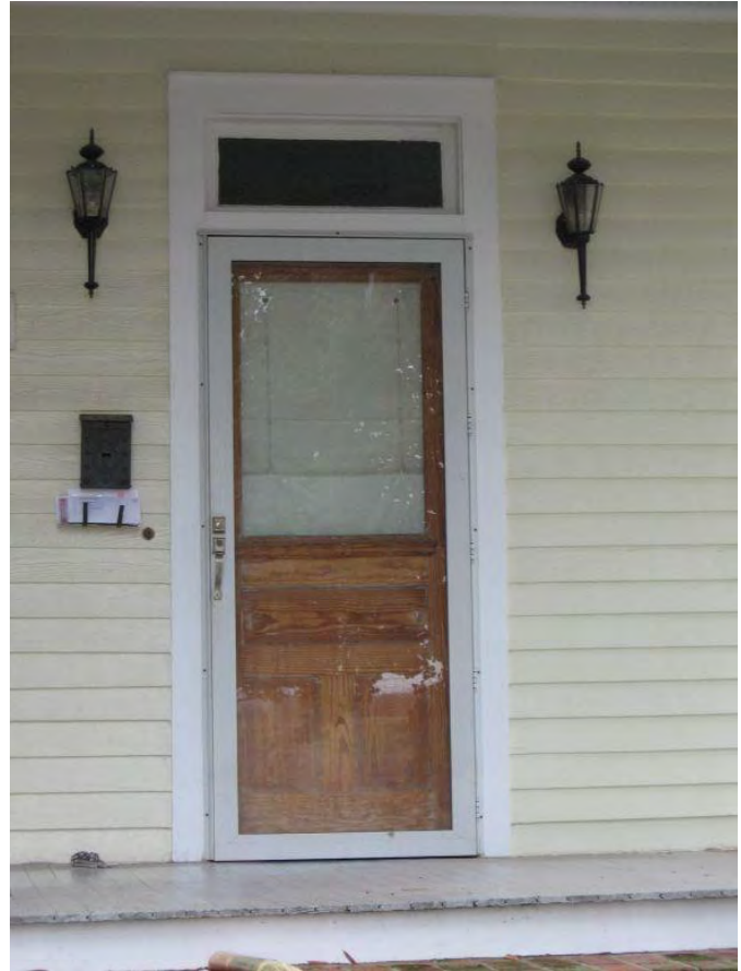
Example of an appropriate storm door which is full-view and the historic door is visible behind it.
