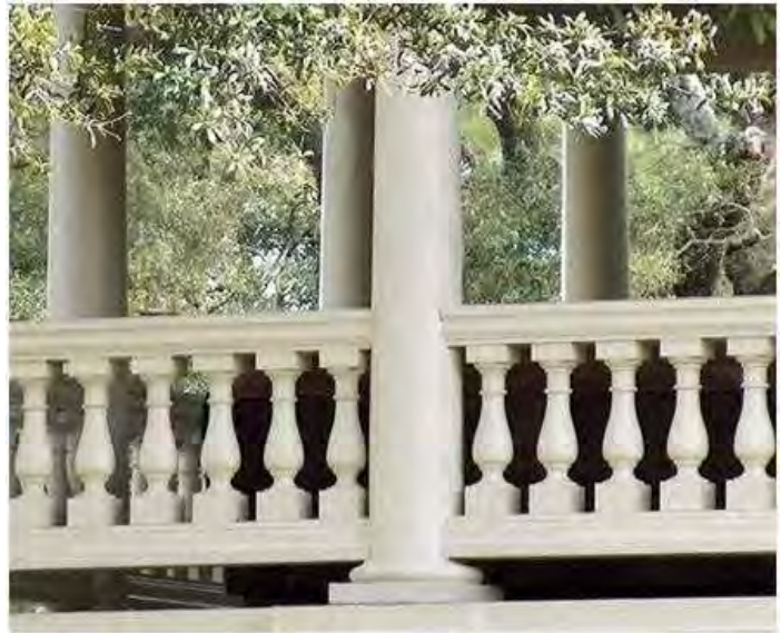
Fiberglass columns and railings as shown above may be appropriate for dwellings when the original columns are no longer extant or if repair is not possible.
