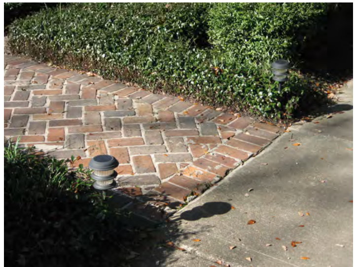
The use of solar powered footlights along walkways is an appropriate method for exterior lighting as shown above.
