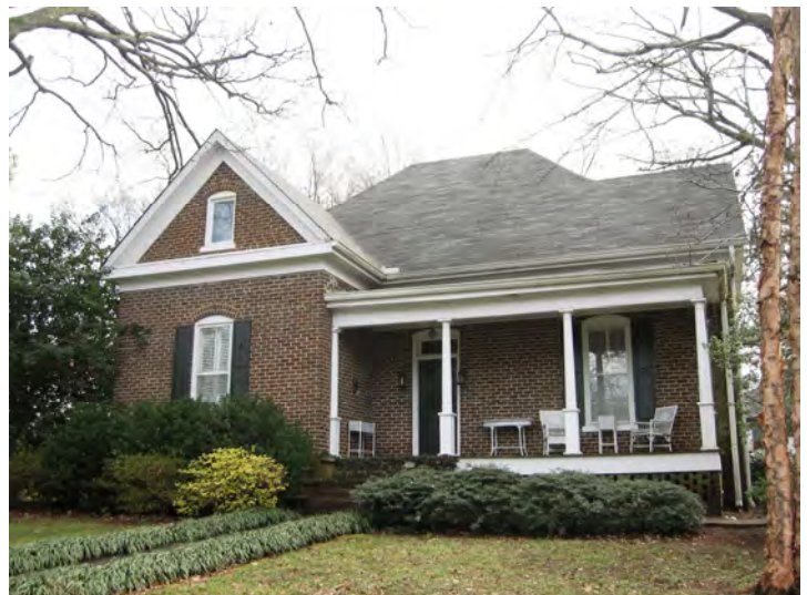
The gabled ell plan refers to the roof form of this type of vernacular design. Altering the roof shape of such a dwelling would compromise the original plan (505 Ingleside Avenue).
