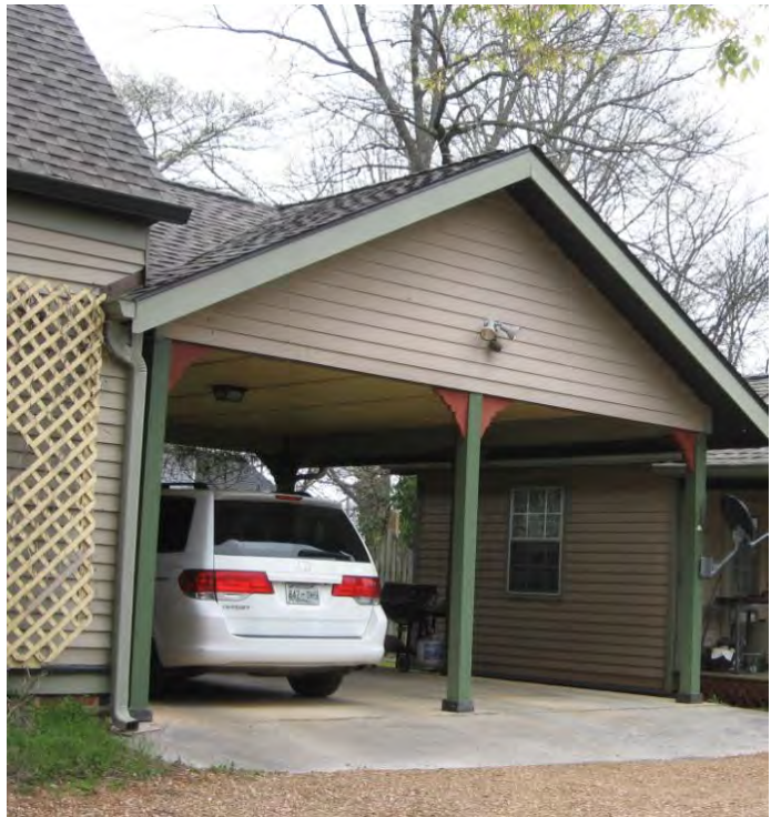
This carport is appropriately designed at the rear elevation of the dwelling and it is not readily visible from the street (419 N. Madison Avenue).
