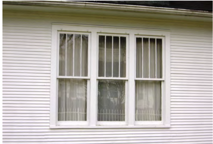
Original four-over-one, vertical-light, wood-sash windows at 504 Ingleside Avenue.
