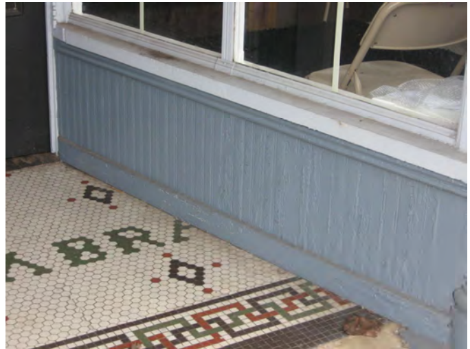
The frame bulkhead at 118 N. Jackson Street (above) and the glazed-tile bulkhead at 2 N. White Street (below) are examples of storefront surfaces that contribute to a varied texture in the commercial streetscape.
