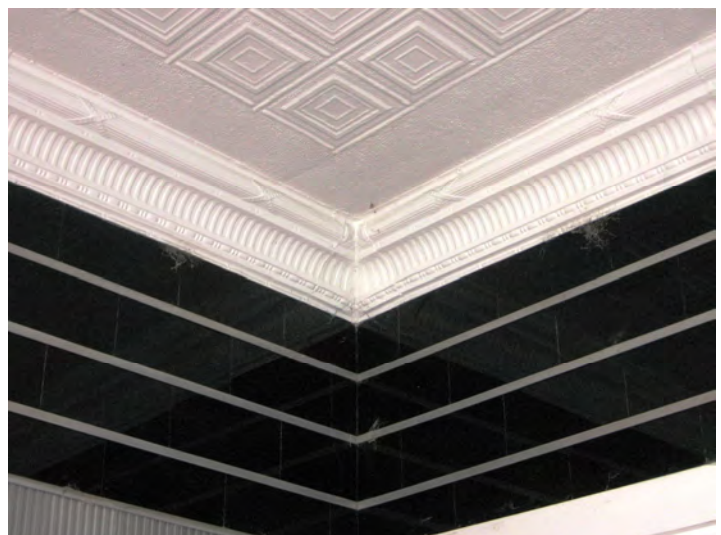
The marble paneled storefront at 2 E. Washington Avenue (above) and the Carrara glass accent courses below a pressed metal ceiling at 4 E. Washington Avenue (below) are examples of storefront surfaces that should be preserved.
